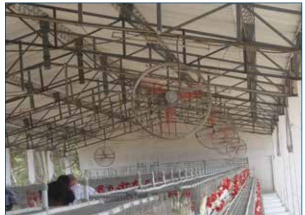
Figure 4. Stir fans and foggers increase air velocity within the house and create a cooling effect.
