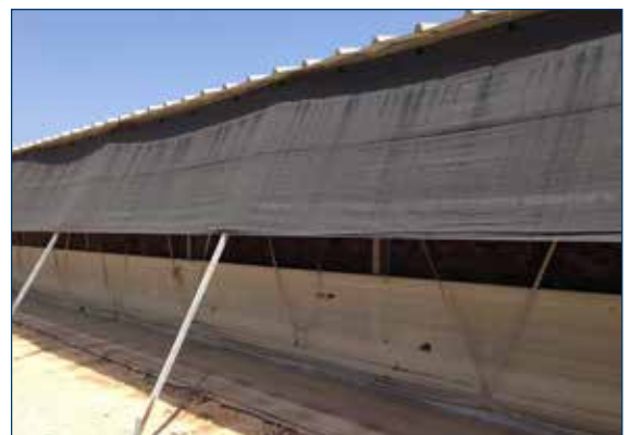
Figure 9. Porous window shades block direct sunlight from entering the house, but allow air to pass through.
