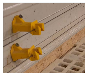
Figure 11. Electrified deterrent wire placed along the perimeter walls and pen partitions.
