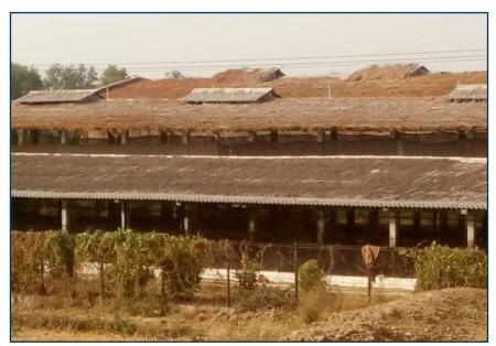
Thatching material (straw or grasses) will reduce heat radiating through the roof.
