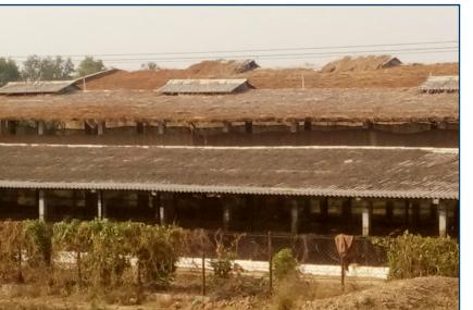
Thatching material (straw or grasses) will reduce heat radiating through the roof.
