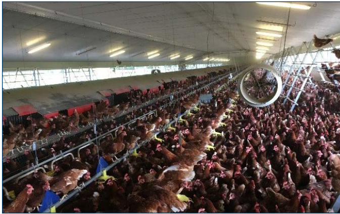
Figure 5. A natural ventilated house with circulatory fans.
